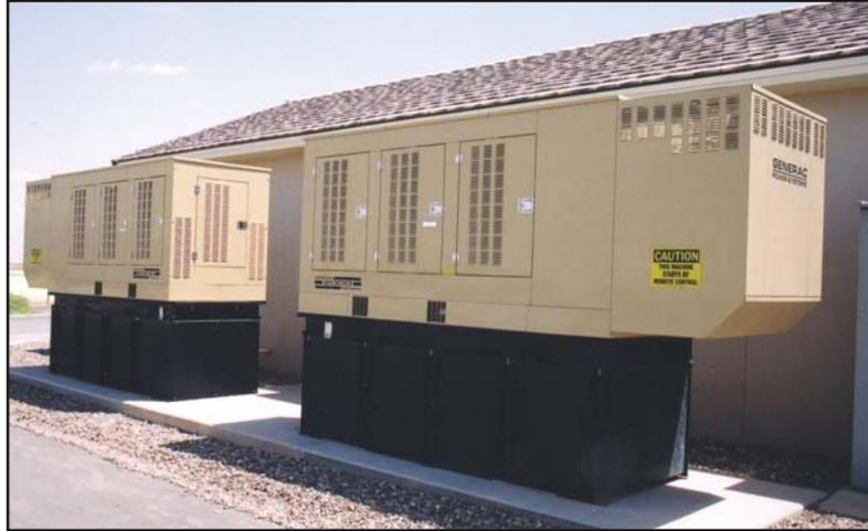
*A pair of 400 kW gensets provide backup power for a wastewater treatment facility.*
